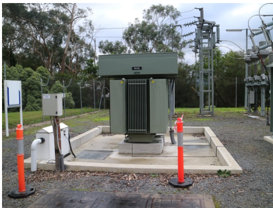
Photos (Left to Right): Arc Suppression Coil, GFN control panels, GFN Inverter
