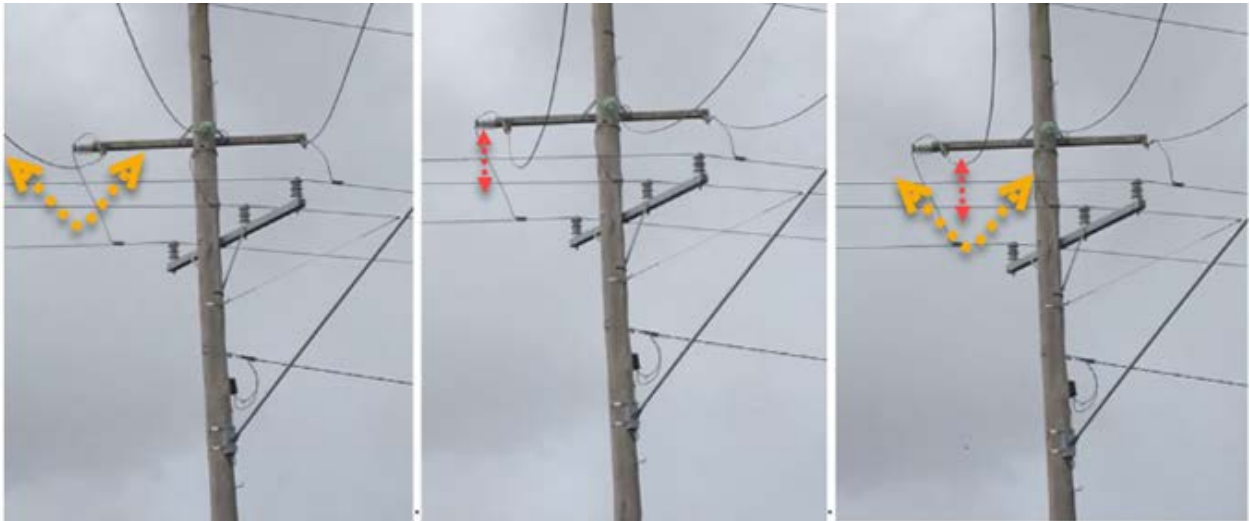
Figure 8: video stills showing the range of conductor movement (horizontal and vertical)
