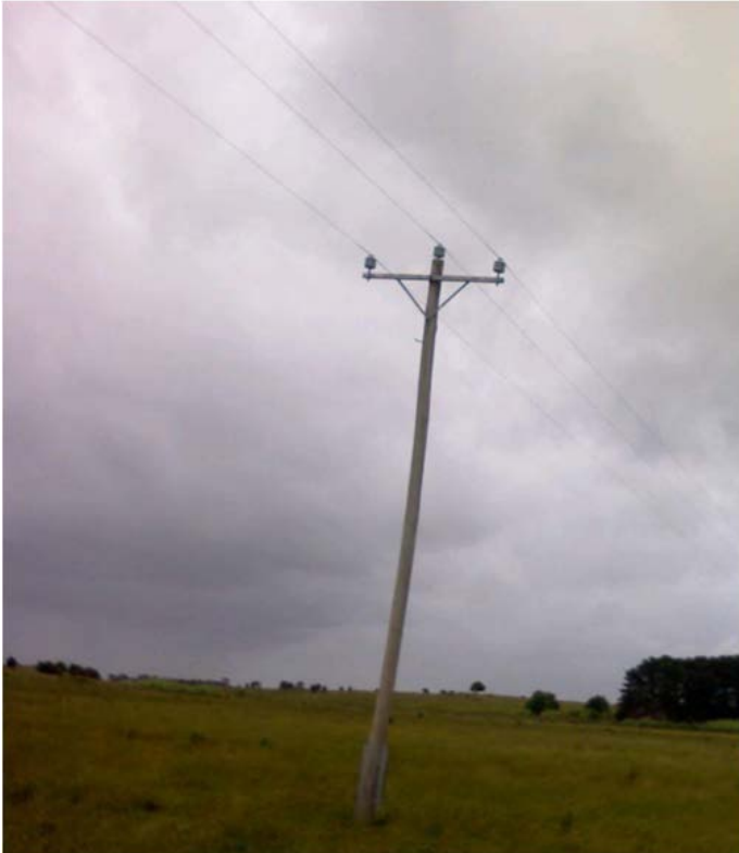
Figure 2 Pole 4 (taken December 5 2012)
