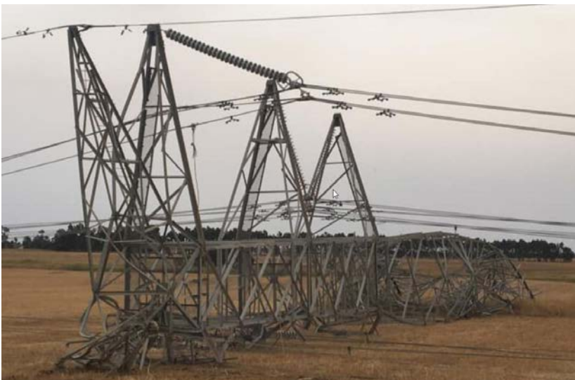
Figure 4 - One of the collapsed towers
